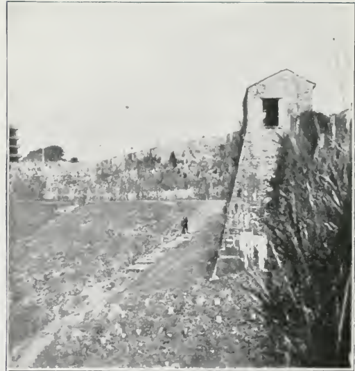
Old Wall, Canton (now demolished)
